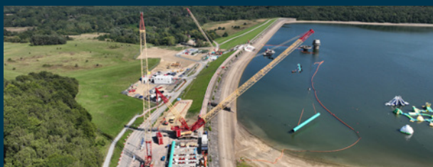
Image: CMDP+ Successful lift of three 29-tonne syphon pipes in August 2025 at Bewl Reservoir operated by Southern Water. We're working as part of the CMDP+ joint venture.
