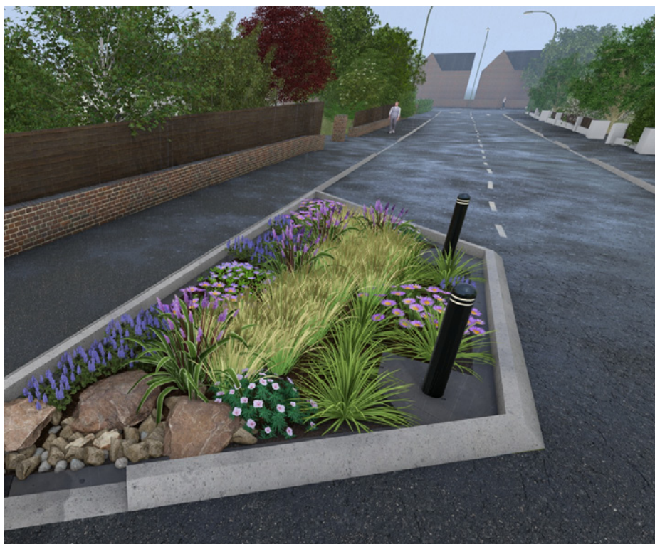
A surface water separation scheme, like a rain garden on a public highway, is one example of the nature-based solutions Tetra Tech is delivering with United Utilities
