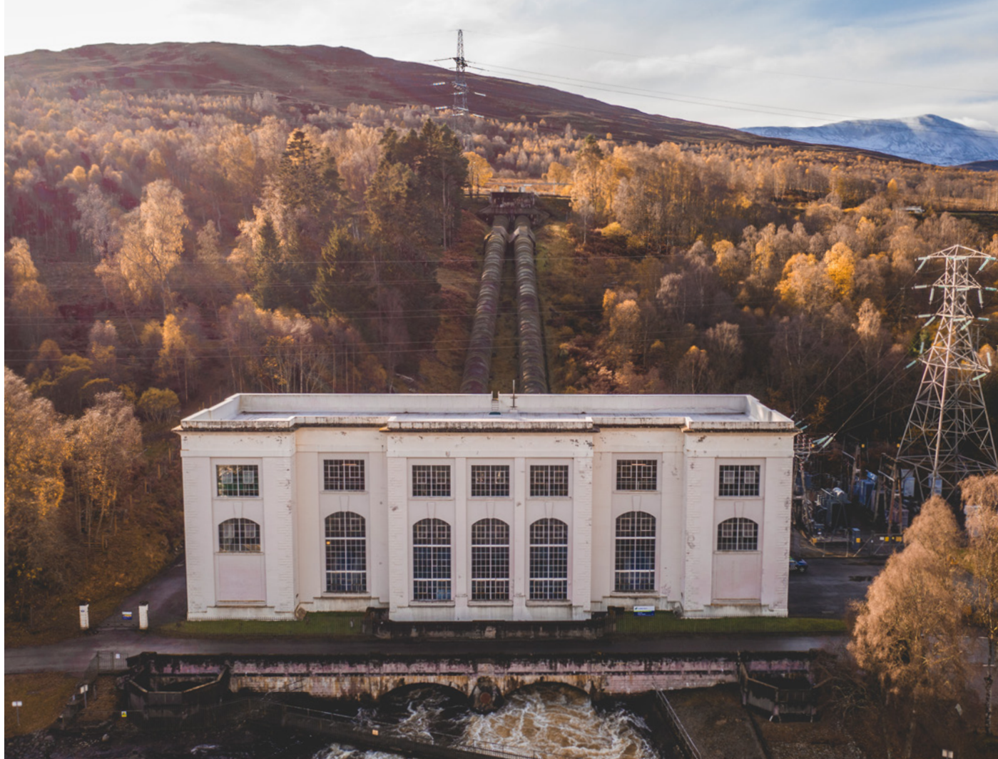
Tummel Bridge Power Station
