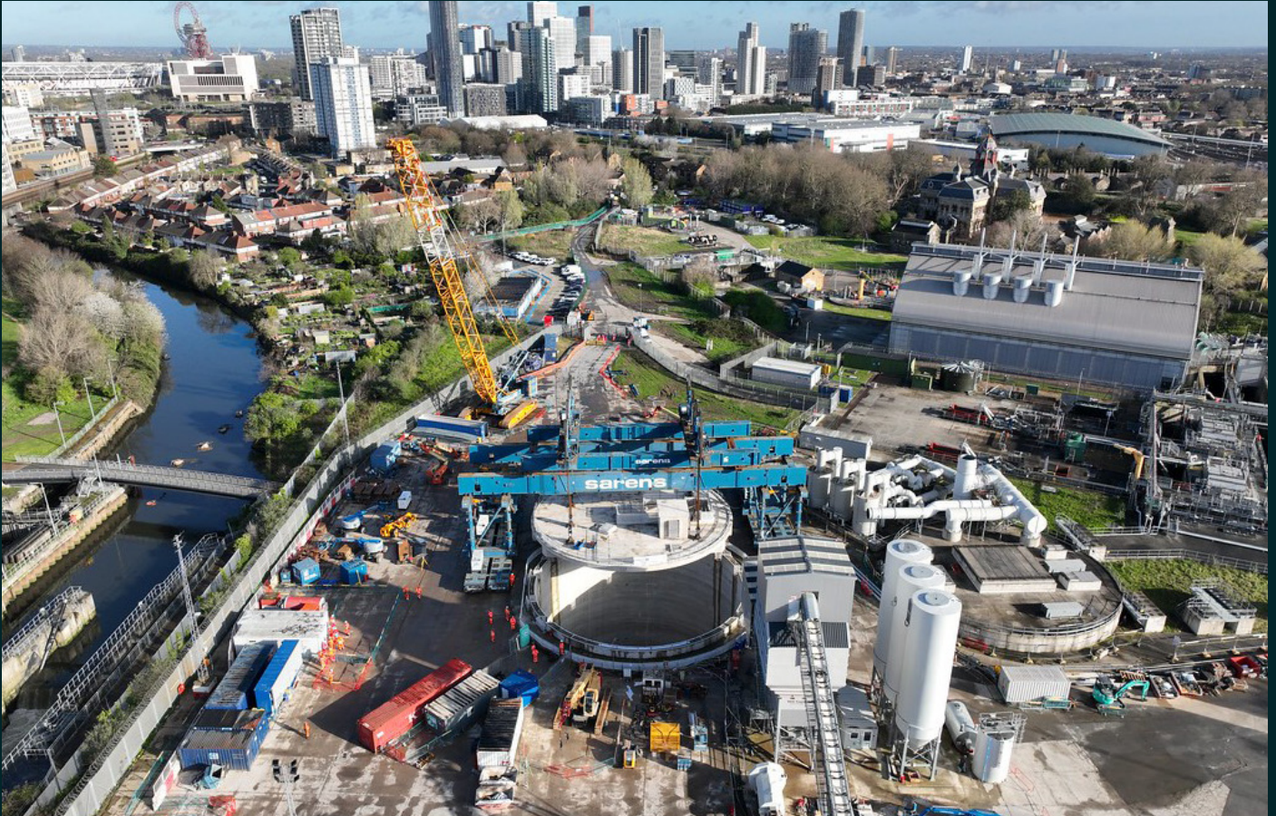
Concrete 'lid' lifted into place over the shaft at Abbey Mills Pumping Station in Stratford, marking completion of underground construction in March 2024
