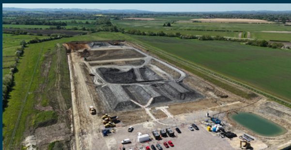
Image: Costain An image of the clay compaction trial site from May 2025 in Abingdon, Oxfordshire, to inform the design of SESRO.
