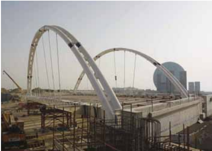
Al Raha construction work underway
